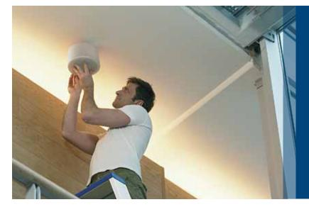
In situations where it is not possible to flush-mount a speaker – for instance, on hard surface ceilings – a stylish Surface Mounting Box makes installation easy and elegant.
