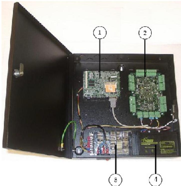
**Figure 4.4** An AEC2.1 access controller
