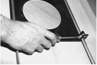
Figure 9.32: Tighten Bracket Securing Screw
