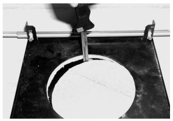
Figure 9.31: Cut Hole in Ceiling Tile
