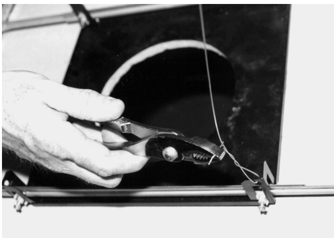
Figure 7.4: Secure Bracket Assembly
